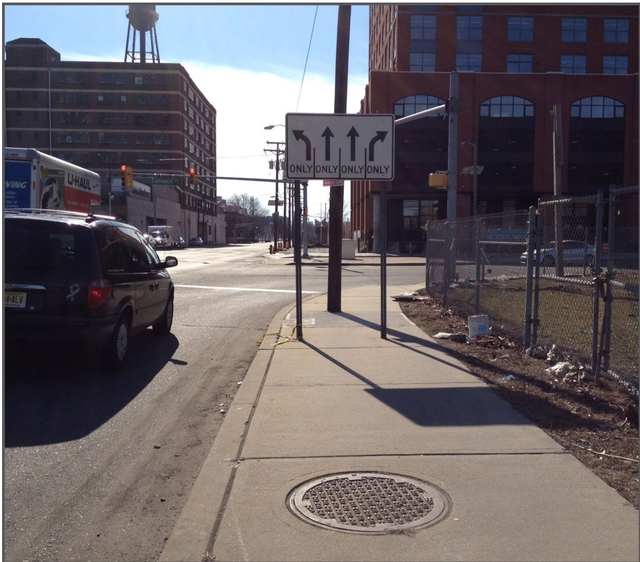
Grove Street and 18th Street intersection crosswalk does not line up with the curb ramp. Image Source: Ben Rosenblatt
