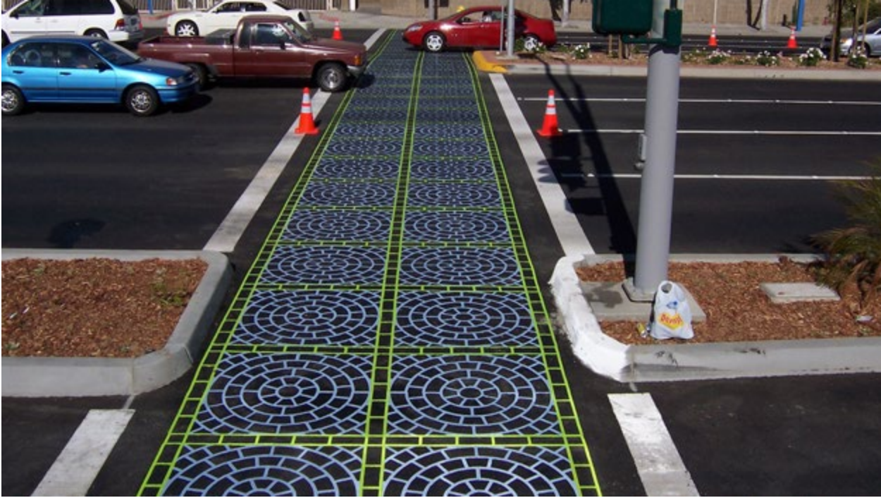
Crosswalk with high visibility thermoplastic markings
