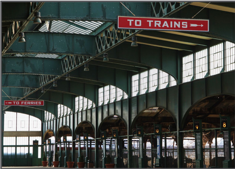
Interior of the CRRNJ Terminal. Image courtesy of wikipedia.com ©2013
