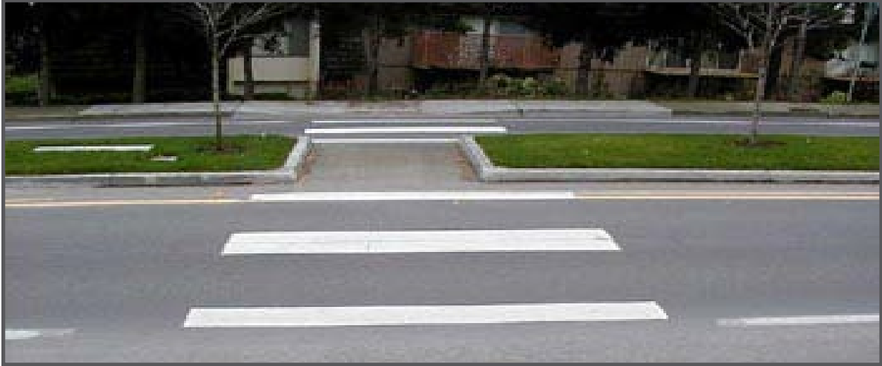
Pedestrian medians shorten crossing distances and provide refuge between travel lanes.
