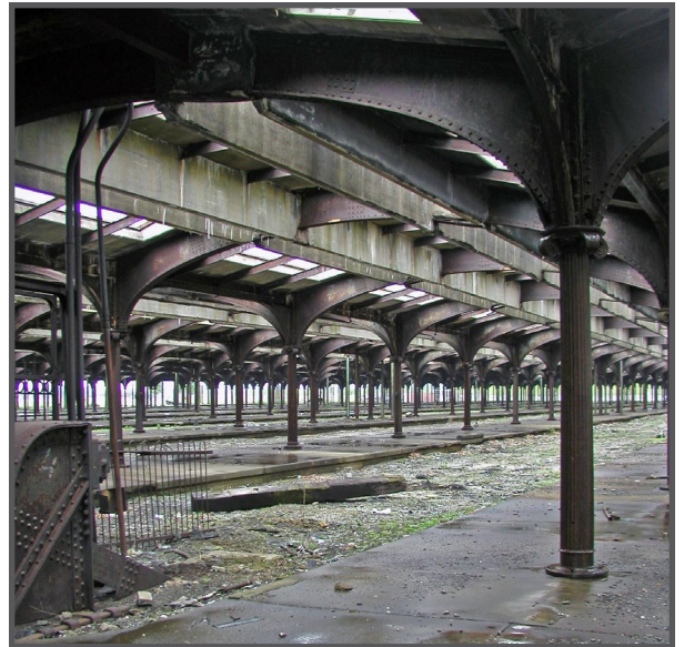
The multi-track train shed at the CRRNJ Terminal Image courtesy of wikipedia.com ©2013
